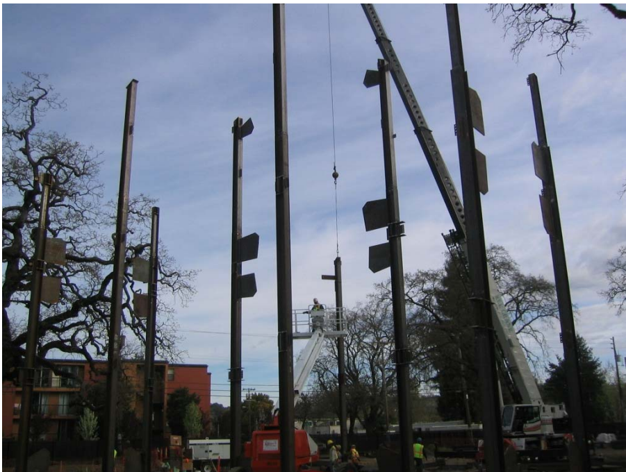
Left: Erection of steel columns by use of mobile crane
