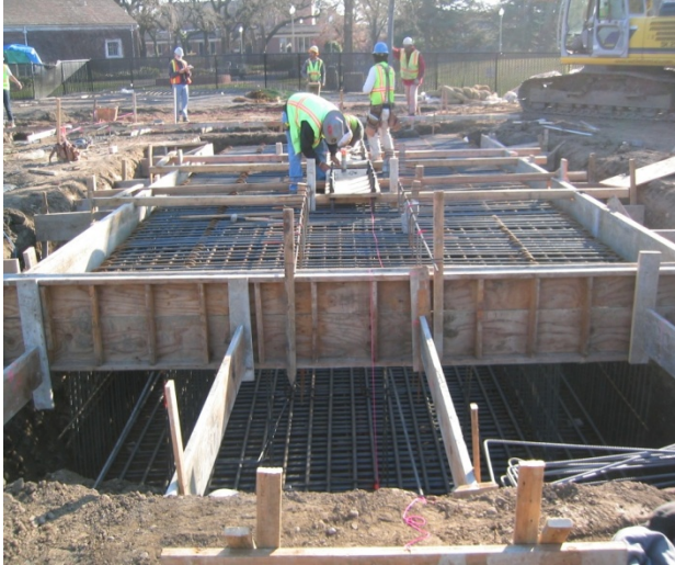
Left: workers placing formwork for an early concrete pour
